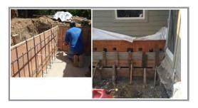
In some existing foundation situations, the structural engineer will recommend that portions of the foundation be removed and replaced with stronger foundations, or better foundation connections. This type of work is intended to gain rigidity in the foundation and lessen the impact on the structure of differential soil movement within the active zone. Underpinning and
