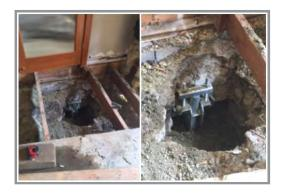
Similar foundation repair, underpinning and the use of adjustable posts within the footprint of a building, can be called for in areas that have settled or moved.
