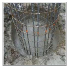
hydraulically driven or drilled deep into the ground beneath the building, beneath the expansive and the active soil zone into what a soil engineer has determined is the likely level of competent load-bearing strata, and then down a specified number of feet further into the earth. Because of the installation methods used in each method, steel piers are sometimes less intrusive, less costly and quicker to install than drilled concrete piers.
